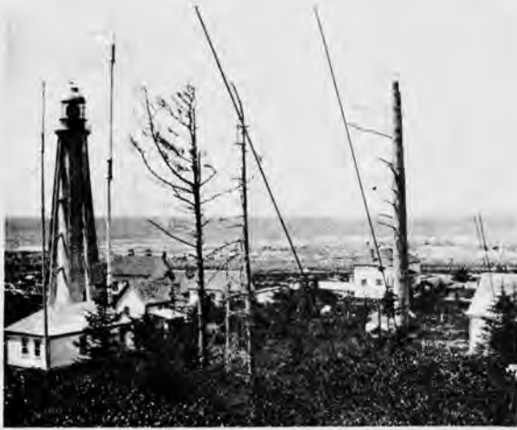
Estevan light, with cluster of wireless buildings and aerial poles.
